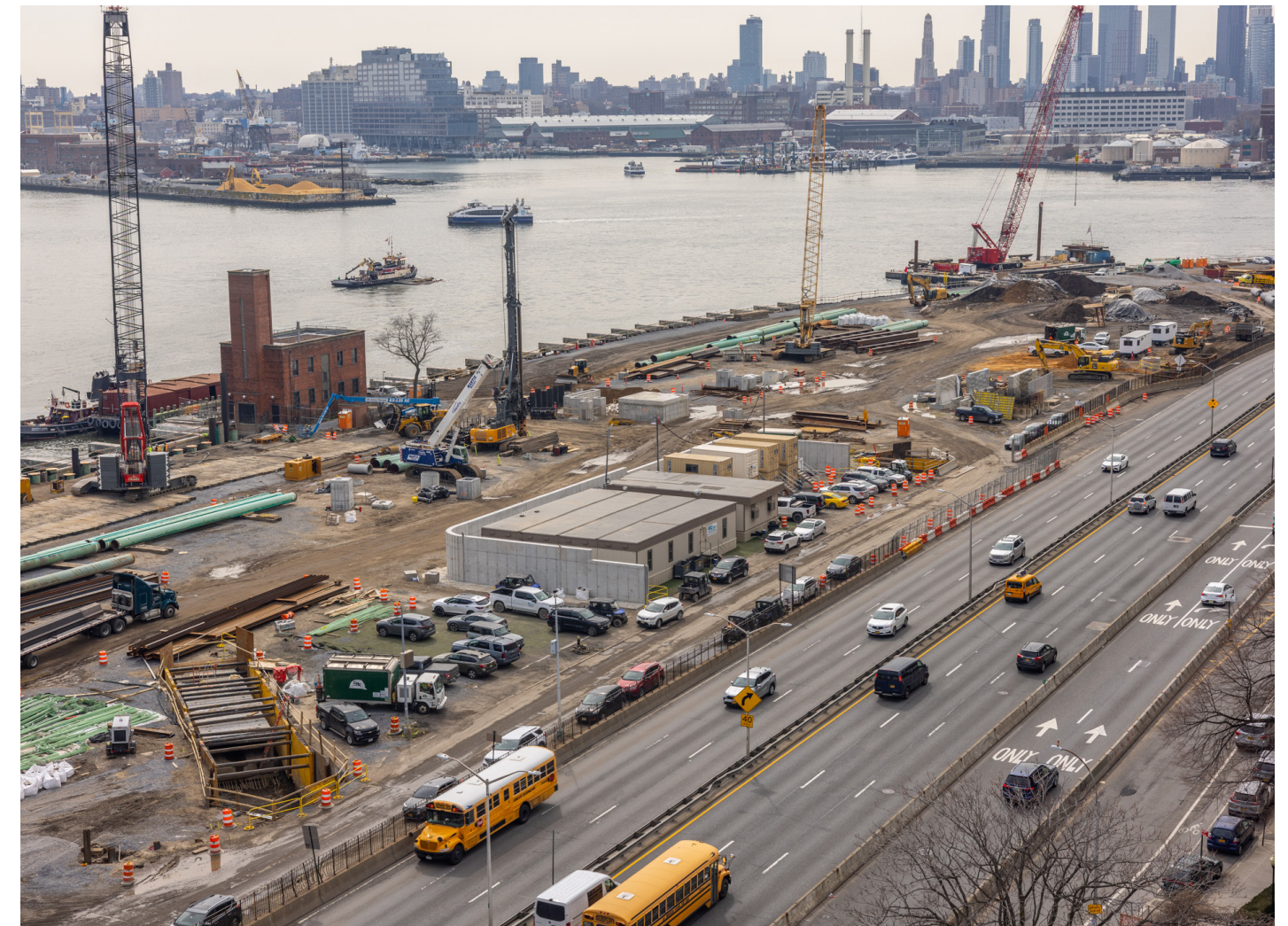
East Side Coastal Resiliency, project area 1 under construction, Spring 2024
