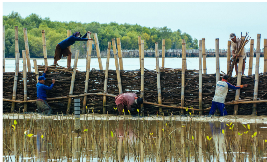
Construction of Permeable structures in Demak Indonesia
