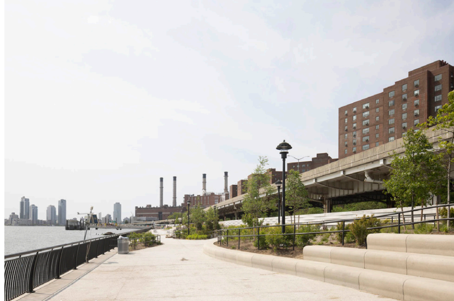
East Side Coastal Resiliency, project area 2 nearly completed
